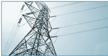
Low, Medium & High Voltage Aerial Lines Installation
