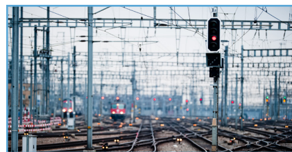
Aerial & Underground Railway Lines Installation
