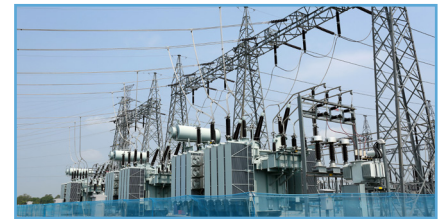
High Voltage Electrical Substations Installation
