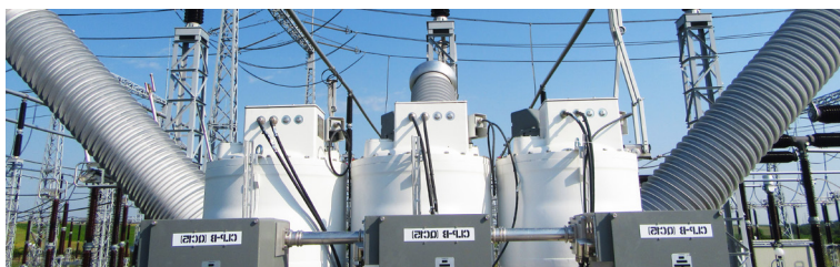
400kV Mobile GIS Substation Bradu & Sibiu
