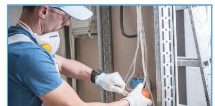
Electrical Appliances Installation
