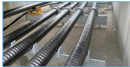
Low, Medium & High Voltage Underground Lines Installation
