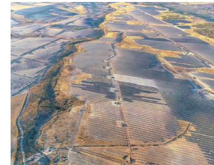
Nuñez de Balboa Power Plant Spain System Capacity: 500 MW (Suntech Supplied 100 MW)
