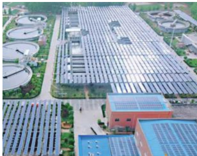
Zhongyuan EP Rooftop Project China System Capacity: 27 MW
