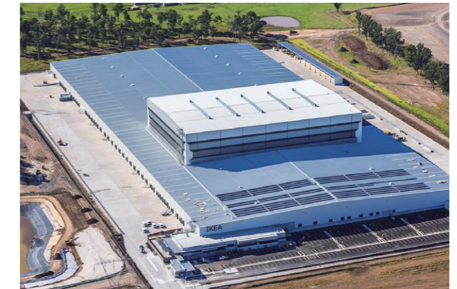
IKEA Rooftop Project Australia System Capacity: 384 KW
