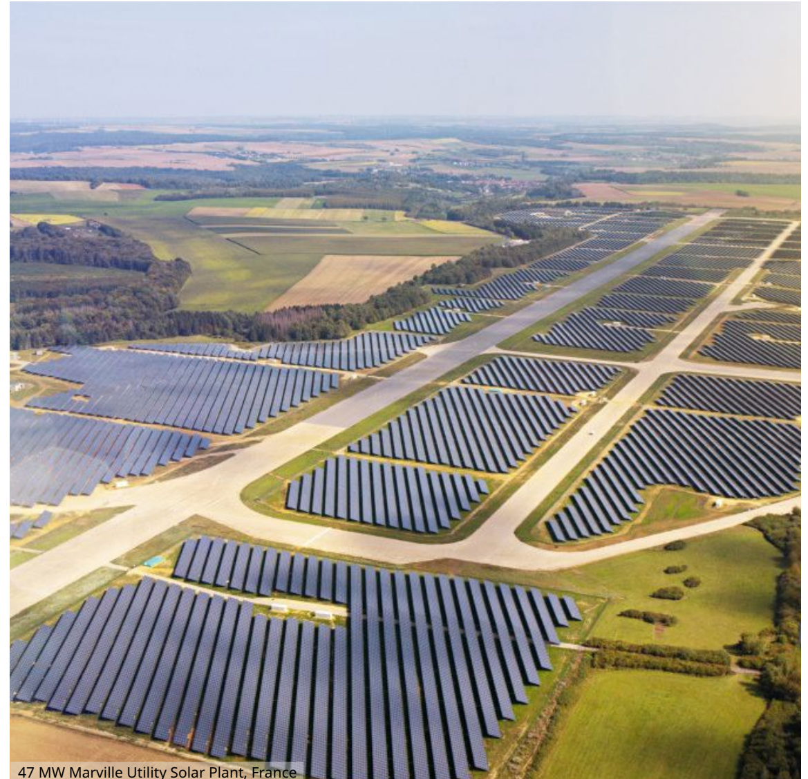
47 MW Marville Utility Solar Plant, France
