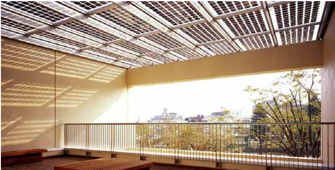
BIPV Project Kowa Elementary School
