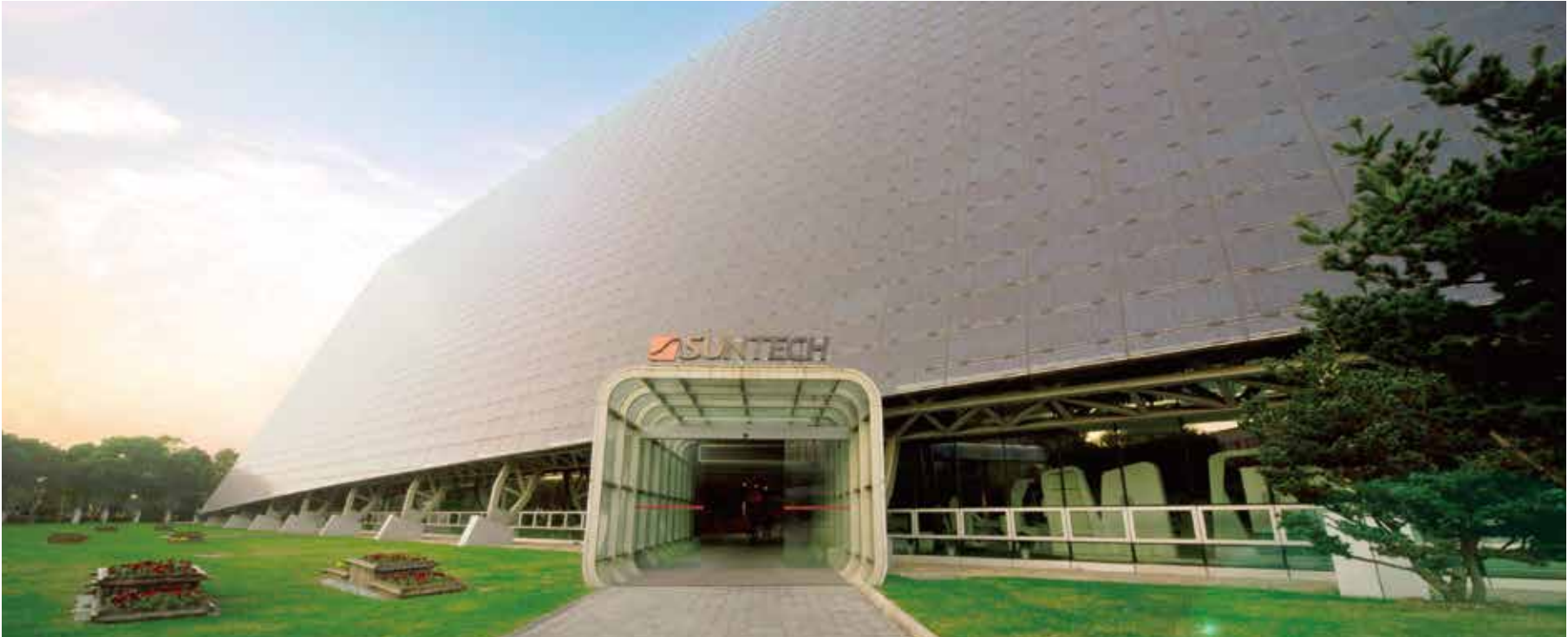
HQ Building BIPV Project Suntech Green Energy
