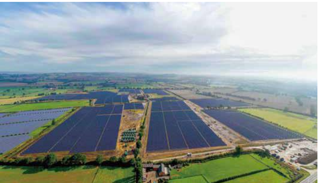
Britain 34.7 MW York Power Plant Project
