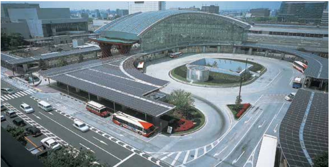
Kanazawa Bus Station BIPV Project
